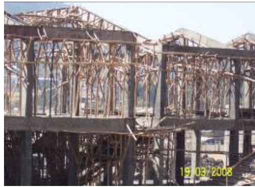
Figure 4. Eucalypt woods for transmission poles and construction poles and posts in Ethiopia (Photo by Mulugeta Lemenih)
