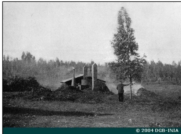
Fig.5. 1928 Sierra Cabello (Huelva). E. globulus oil boiler. (Montero et al. 2007)
